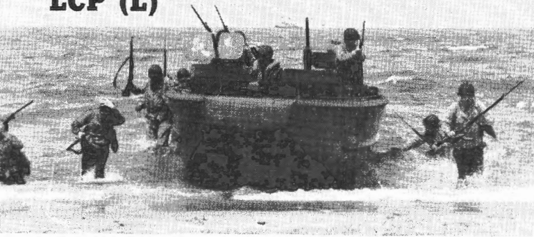
Loaded LCP(L) beaching its troops. Debarkation has been improved by the addition of a bow ramp (LCP(R)).
