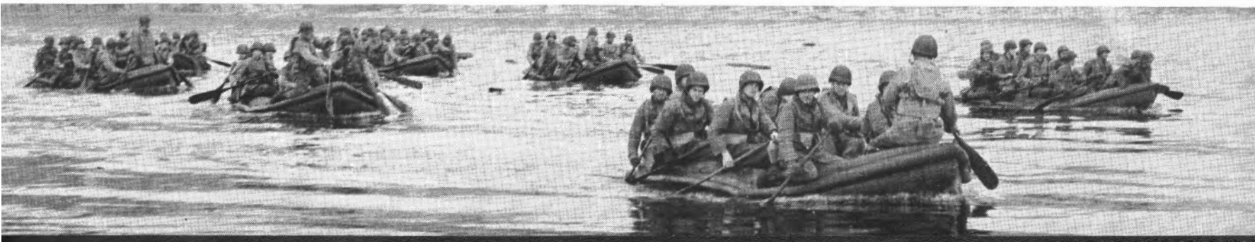
▼ LCR(L)'s in operation; A light machine gun may be mounted in bow position.
