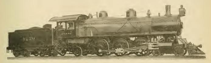
POWERFUL NEW PASSENGER LOCOMOTIVE.—ATCHISON, TOPEKA & SANTE FE RAILWAY. 4-6-2 TYPE. BUILT BY BALDWIN LOCOMOTIVE WORKS.
