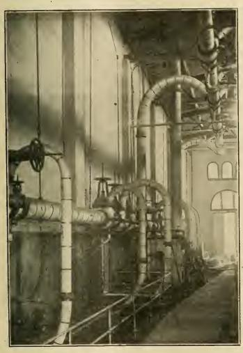
VIEW OF STEAM PIPING SHOWING SWING METHOD OF SUSPENSION
