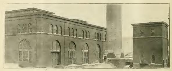
SOUTHWEST CORNER OF POWER-HOUSE, SHOWING STACK AND DUMPING ASH-TOWER AT RIGHT.
