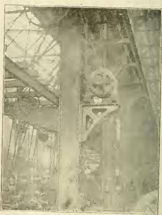
CLOSE VIEW OF MOTOR—SHOWING BRACKET SUPPORTS—EAST SIDE OF MACHINE SHOP BAY,
