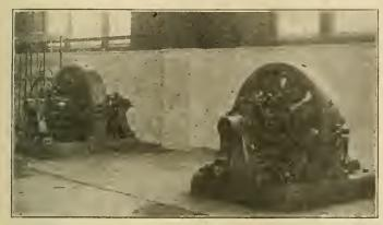
THE 150-K.W. ROTARY CONVERTORS SUPPLYING THE CRANE AND OTHER DIRECT-CURRENT MOTORS.
