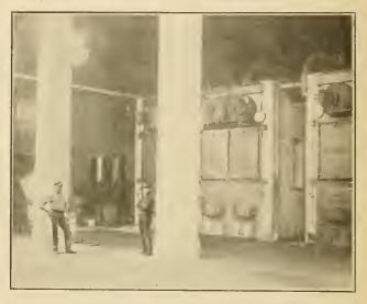
MEW IN THE BOILER ROOM, SHOWING CONCRETE PIER CONSTRUCTION.—BABCOCK & WILCOX BOILERS.
