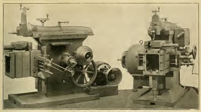
HIGH-SPEED BELTED DRIVE UPON A 20-IN CRANK SHAPER.—JANTZ & LEIST MULTIPLE-VOLTAGE VARIABLE-SPEED DRIVE. -MOTOR. LOCK ELECTRIC MANUFACTURING COMPANY. MOTOR-DRIVEN SHAPERS.—CINCINNATI SHAPER COMPANY.
