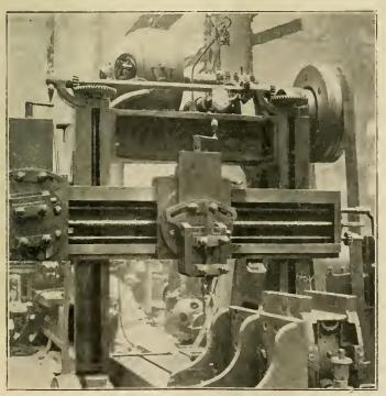
36-in. x 36-in. x 10-ft. planer.—pond machine tool co. fly-wheel drive from a  $7\,^{\rm h_2}$ -h.p. multiple-voltage crocker-wheeler motor. SPECIAL
