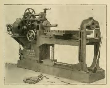
$60\text{-}\mathrm{Inch}$  horizontal boring and drilling machine.—Niles tool works co. Driven by a 5-h.p. multiple-voltage c.-w. motor.
