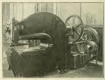
36-in. throat no. 4 single punch.—long & allstater company. Driven by a 3-h.p. CONSTANT-SPEED C.-W. MOTOR.
