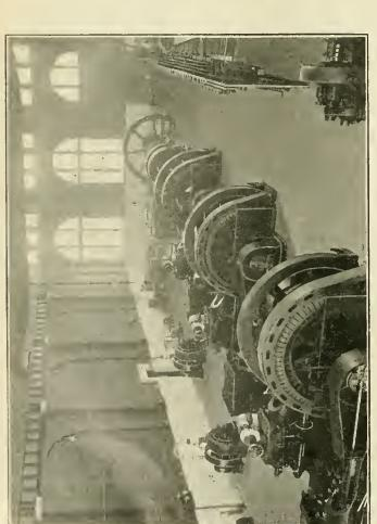
VIEW OF ENGINE-ROOM PROM NORTHWEST CORNER, SHOWING GENERATOR AND EXCITER UNITS.
