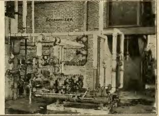
VIEW OF THE BOILERS, SHOWING TRAVELING LINK GRATES, FEED-WATER HEATER AND PUMP GOVERNOR.
