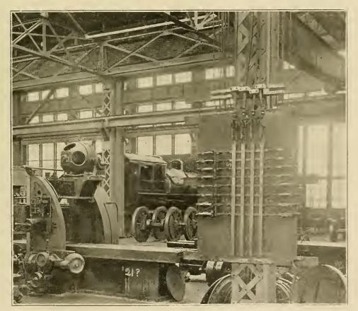
VIEW OF A TYPICAL TABLET BOARD IN THE MACHINE SHOP, FROM WHICH FOUR MOTOR CIRCUITS ARE FED.
