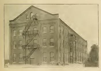
CARPENTER-SHOP BUILDING, SHOWING OUTSIDE STEEL CONSTRUCTION FOR ELEVATOR SERVING THE PATTERN LOFTS.
