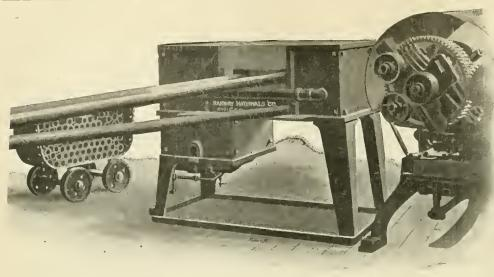
VIEW OF THE FLUE WELDING FURNACE IN PLACE. THE OIL FURNACES.—COLLINWOOD SHOPS,
