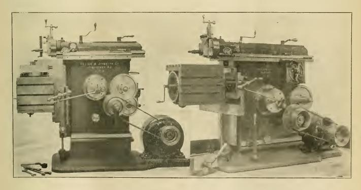
BELTED DRIVES UPON 15-IN. AND 24-IN. UNIVERSAL GRANK-SHAPERS—BUILT BY THE POTTER & JOHNSTON MACHINE COMPANY, CONSTANT-SPEED MOTORS.—GENERAL ELECTRIC COMPANY,
