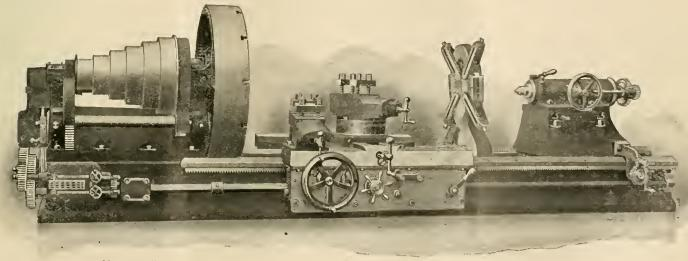
NEW DESIGN OF THE 60-INCH "AMERICAN" LATHE, WITH QUICK CHANGE-GEAR MECHANISM.—AMERICAN TOOL WORKS COMPANY.
