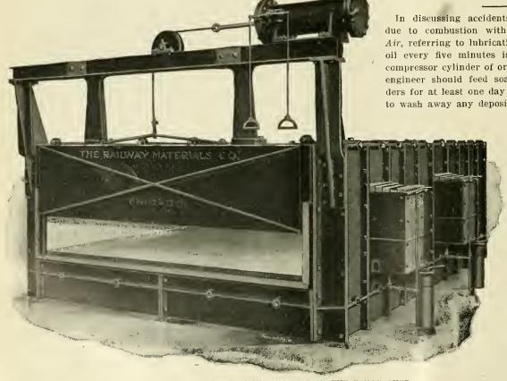
THE LARGE ANNEALING AND FLANGING FURNACE IN THE BOILER SHOP. THE OIL FURNACES. -COLLINWOOD SHOPS.
