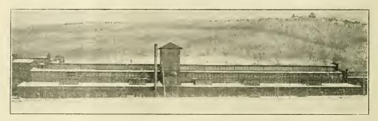
BOILER SHOP, FROM HIGH GROUND TO THE WEST. RIVETING TOWER AT THE CENTER. SHOWS THE LARGE AMOUNT OF GLASS IN ROOF.
