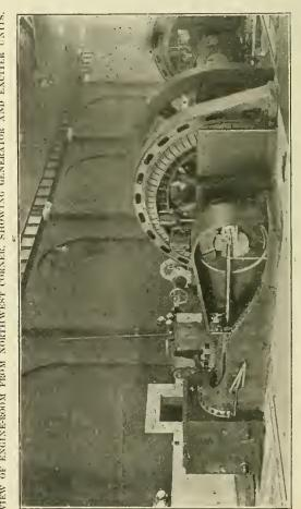
THE 400 KW, GENERAL ELECTRIC TWO-PHASE GENERATOR UNIT. -- 600-H.P. M'INTOSH &
