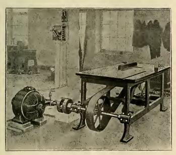
FIG. 3.—A 12-INCH RIP SAW WITH A DIRECT-COUPLED DRIVE FROM A 10-II. P. BACK-GEARED MOTOR.
