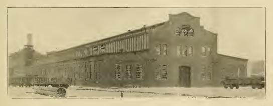
FOUNDRY FROM SOUTHWEST CORNER, SHOWING INSULATOR-RACKS AT GABLE WINDOW FOR OVERHEAD WIRE: SYSTEM.
