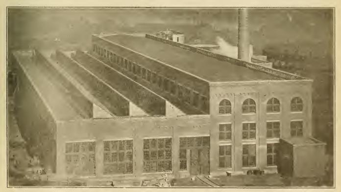
VIEW OF THE MACHINE AND ERECTING SHOP BUILDING FROM THE HILL AT THE WEST SIDE OF THE SHOPS, SHOWING ARRANGEMENT OF SAW TOOTH WIDOWS AND SYMMETRICAL LINES OF CORNICE AND FINISH OF BUILDING.
