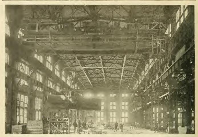
INTERIOR VIEW IN ERECTING SHOP, SHOWING 120-TON CRANE LIFTING A BOILER. SHOWING ALSO HEAVY CHARACTER OF STEEL CONSTRUCTION.
