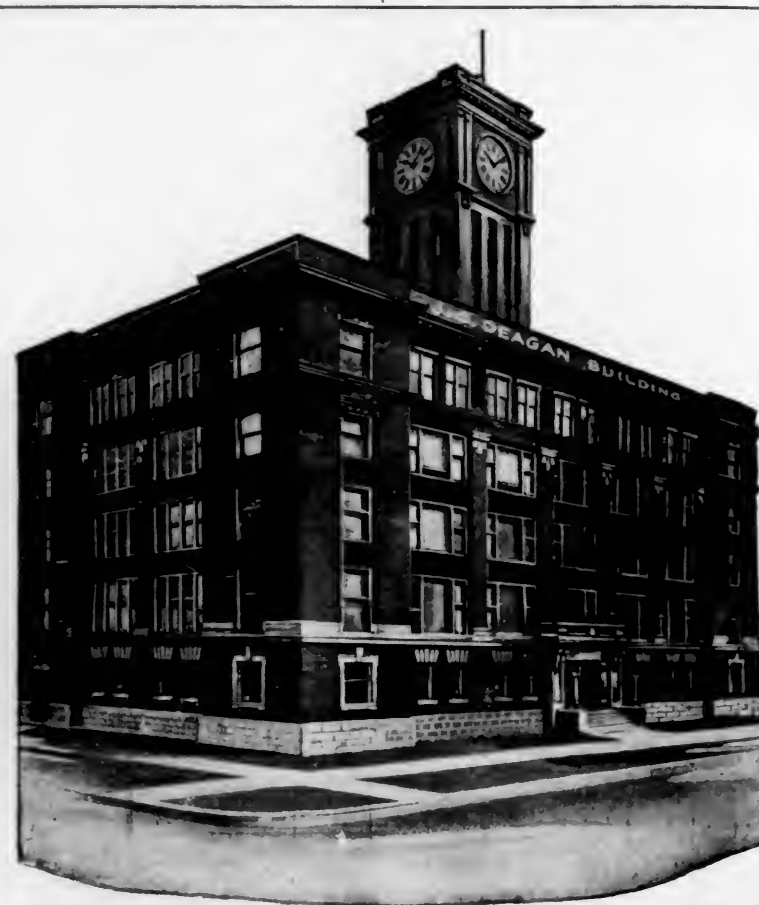
The new home of the J. C. Deagan Musical Bells, located at 1770 Bertrou Avenue, North, Chicago. It is a five-story, 160 feet long by 100 feet wide, made of reinforced concrete, and has a floor area of over 80,000 feet. This building is said to have cost $375,000. Mr. Deagan recently returned from an extended trip of one year through Africa, Asia and Europe in search of the materials for sounding boards and musical woods, etc. It is expected that this enterprising manufacturer will soon have some startling announcements to make pertaining to his line of endeavor.
