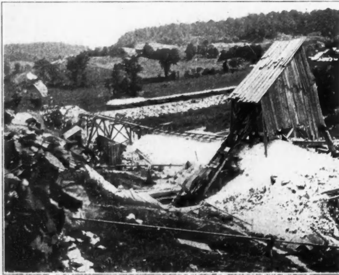
FIG. 1.—ENTRANCE TO MINE NO. 5, TALCVILLE.
